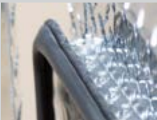
Built-in rain gutter with automotive seal
